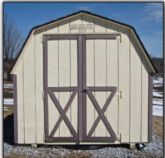
AE - 4 Fire District Storage Shed
