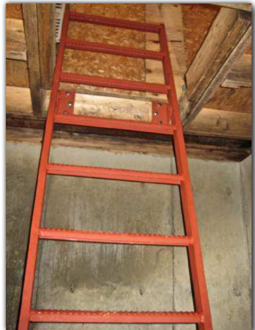
AE - 18 Ladder to Lower Level
