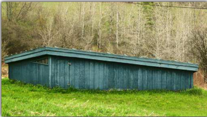
AE - 3 Fire District Spring Collection Box
