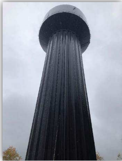
AE- 122 Water Tower
