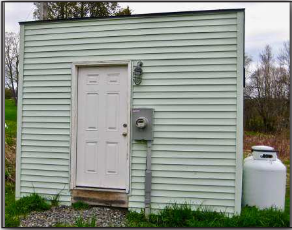
AE - 1 Fire District Pump House
