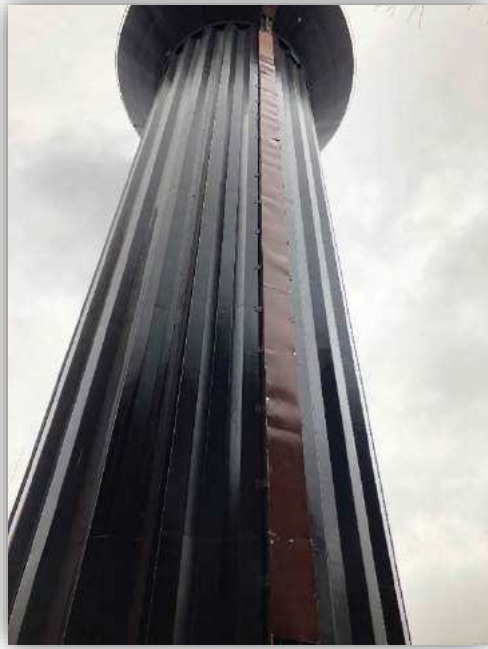
AE- 130 Water Tower
