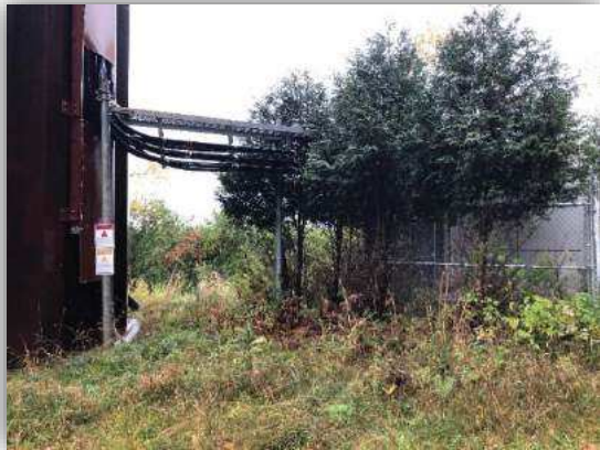
AE- 128 Tower Exterior
