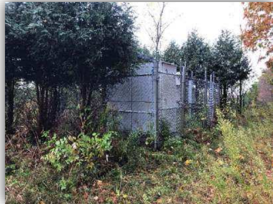
AE- 129 Tower Exterior
