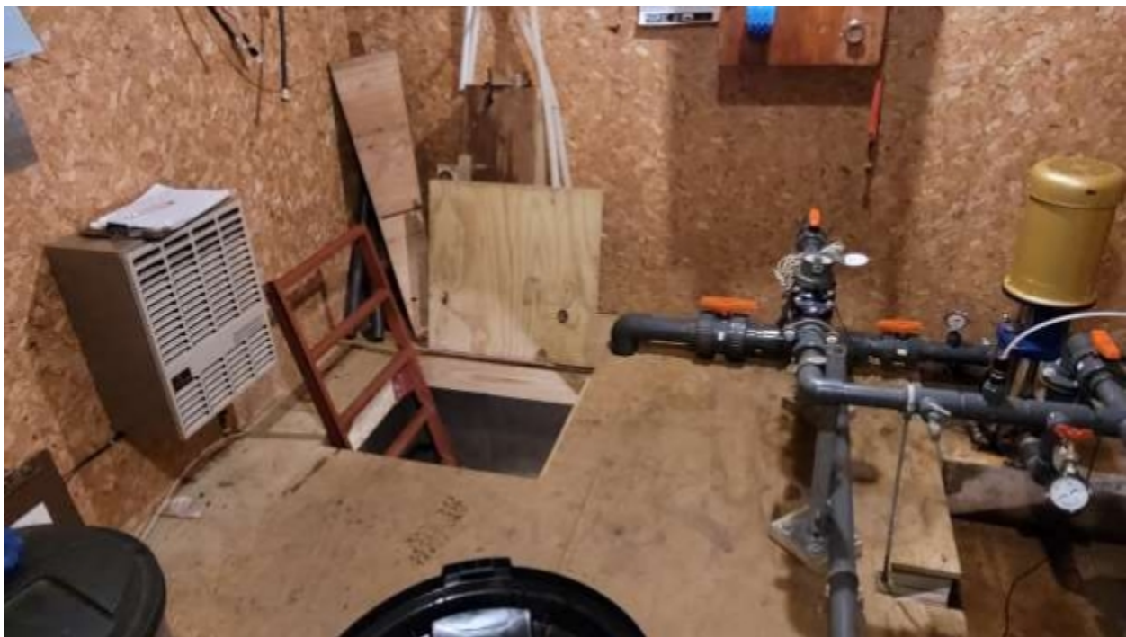
Hatchway and ladder to basement level of Treatment Building
